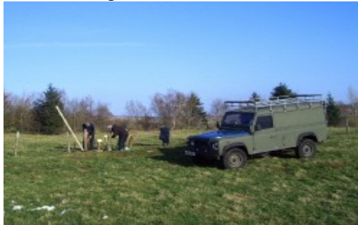
Installing a stile in November sunshine
